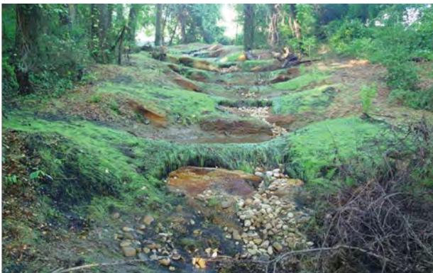
*Figure 4.8-1e. Regenerative Stormwater Conveyance (Photo: Biohabitats, Inc.)*
