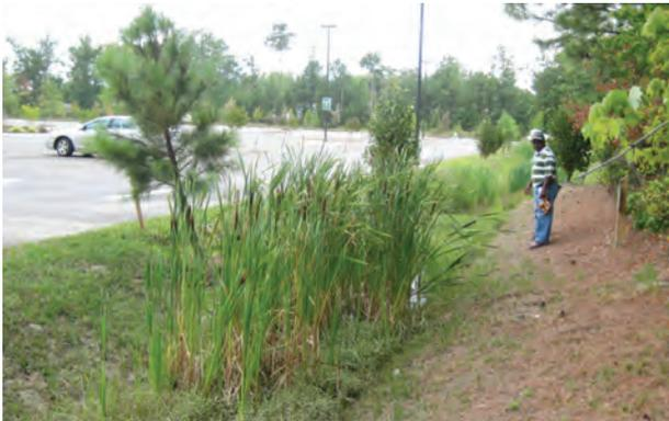
*Figure 4.8-1c. Wet Swale (Photo: CWP)*
