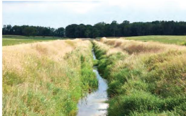
*Figure 4.8-1d. Two-Stage Ditch (Photo: Ohio State University Extension)*
