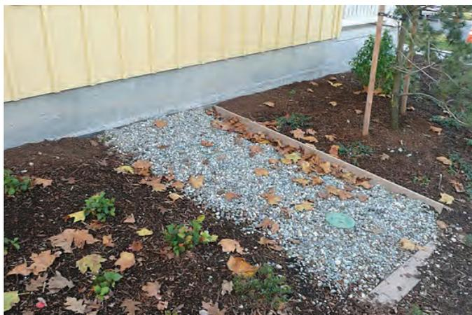
Figure 4.4-3. Infiltration to Treat Roof Runoff (Micro-Scale)
