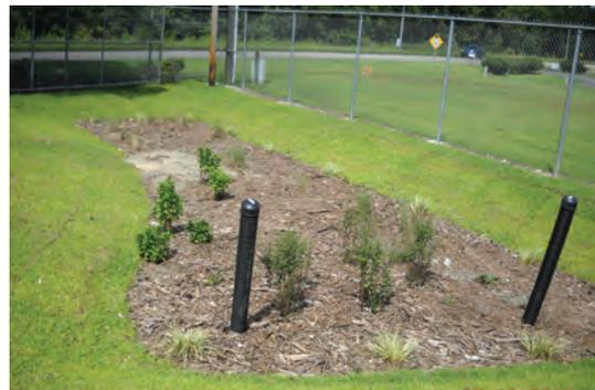
Figure 5.2-2. Bioretention cell at Loris Recycling Center (Photo: Horry County Stormwater Management)
