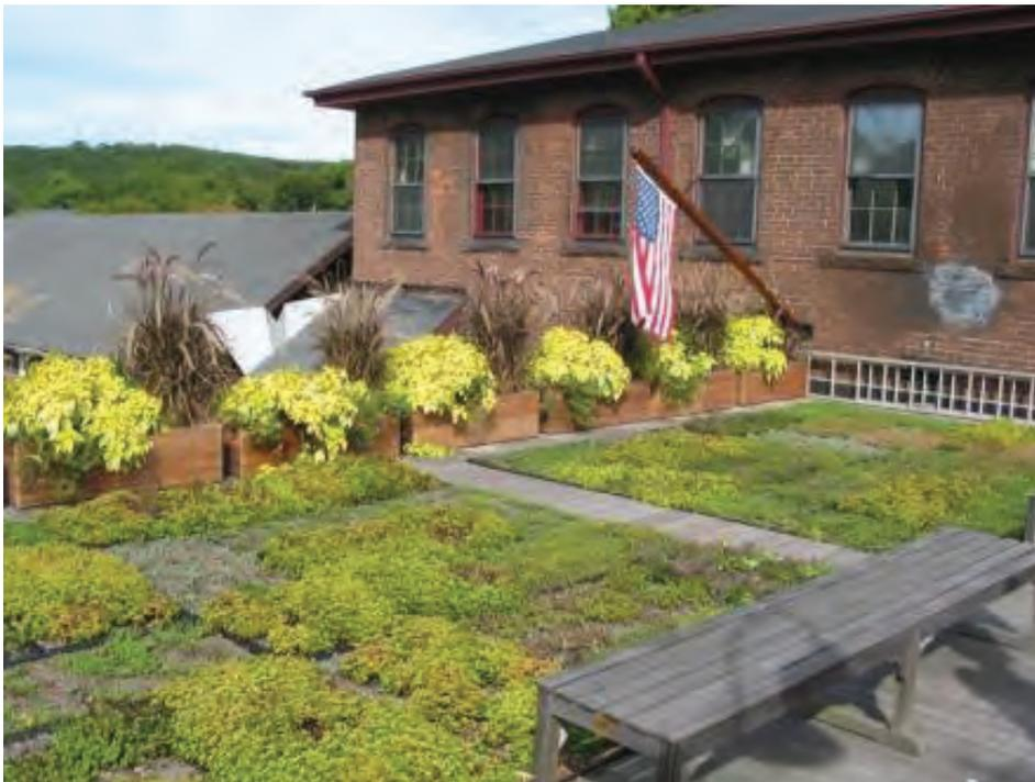
Figure 4.5-1. Green Roof (Photo: Center for Watershed Protection)
