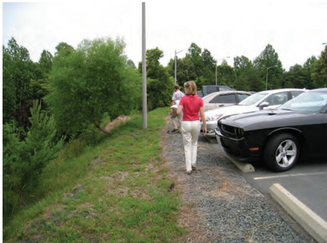
Figure 4.4-2. Infiltration at Edge of Parking Lot
