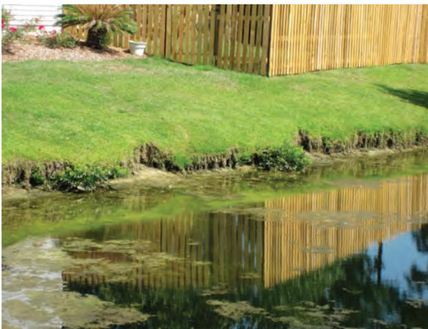
Figure 5.1-2. Bank erosion prior to restoration treatment
