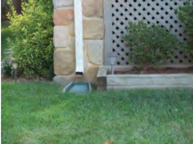
Figure 4.7-1. Simple Rooftop Disconnection
