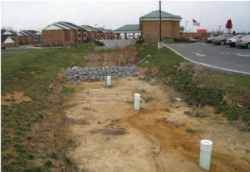
Figure 4.4-8. Infiltration Sand Filter Example (Photo: CWP)
