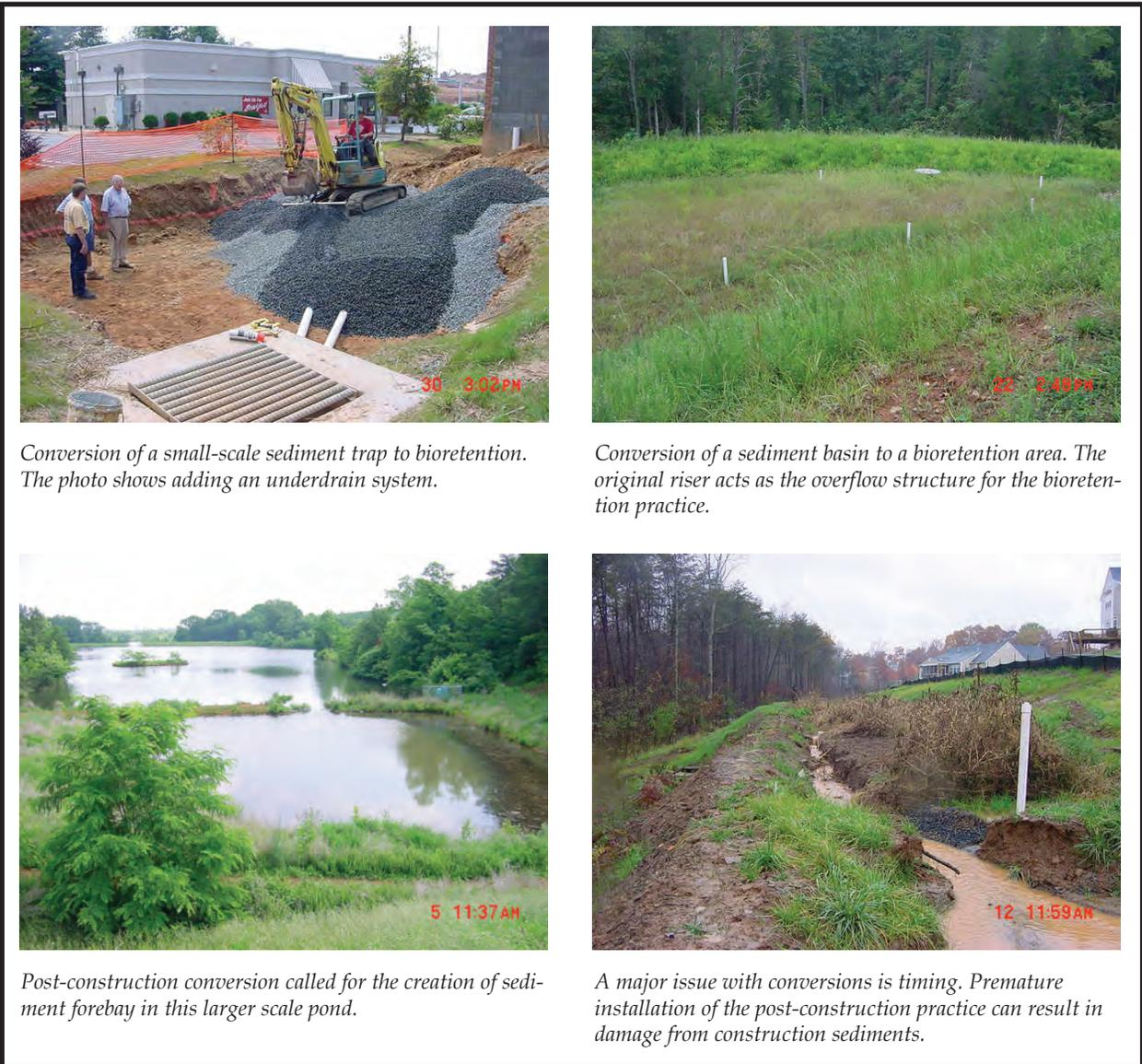
Figure E.3-1. Examples of E&S control practice conversions to post-construction BMPs (Photos: Center for Watershed Protection)
