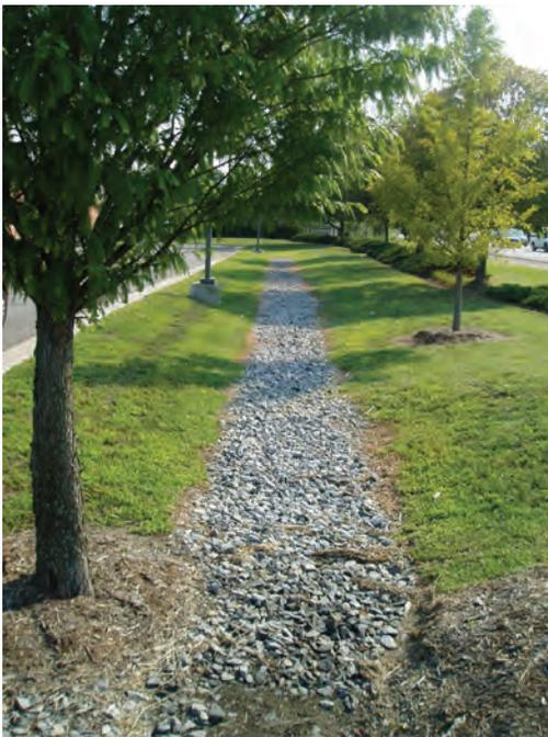
Figure 4.4-1. Infiltration in Median Strip
