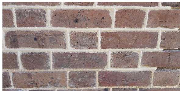
The historic brick façade will be repointed with a "bird's beak" or "double-struck" joint. While uncommon, this joint profile was the original (1888) treatment for the building. This profile helps to visually straighten the slightly irregular brick profiles. Photo above shows the sample panel above existing mortar.
