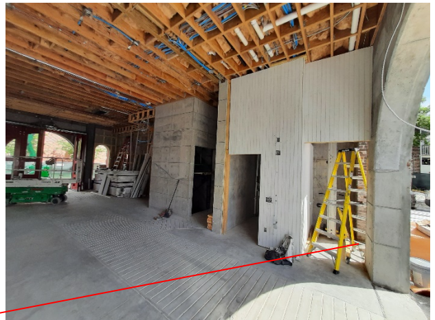
A view of the main apparatus bay (SW corner). The elevator will be in the concrete structure at center, with a passageway to east side. The opening in the beadboard wall leads to a bathroom. The yellow ladder is in the new exit door location.
