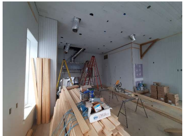
A view from the NE corner on the second floor, in the Day Room and Kitchen area. Beadboard walls & trim are largely complete in this area. The kitchen hood exhaust duct is one of the last mechanical systems to be installed upstairs.
