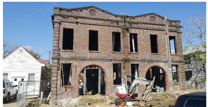
Contractor is 'hopscothing' around the perimeter, constructing pile caps and grade beams in alternate fashion.
