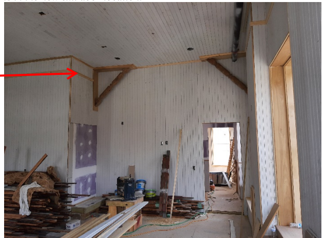
A view from the NE corner on the second floor, in the Day Room and Kitchen area. Beadboard walls & trim are largely complete in this area. Note the historic brackets along the far wall. These decorative elements were once part of the structural center wall that was originally located in this area (see photo left). The new reinforced concrete wall is hidden behind the beadboard.
