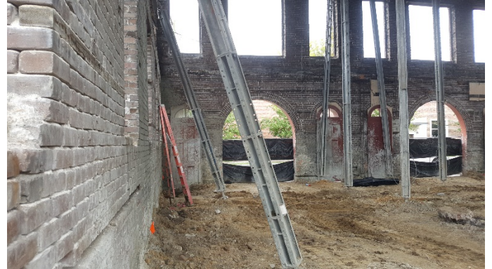
Installation of interior micropiles and temporary shoring complete in this area.
