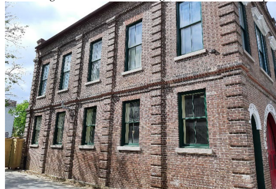
East elevation, viewed from neighbor's driveway. There are 190 'street bolts' for the hurricane protection system hidden in the brick on this elevation .
