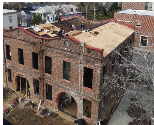
The original terne metal roof has been removed and the existing roof deck repaired before being covered with plywood and ice & water shield. After the brickwork is repaired and new structural system completed, a standing seam copper roof will be installed. View from the historic fire tower on 12.23.2020.
