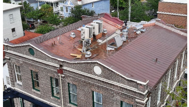
The new copper roof is nearly complete, and the mechanical equipment is being set in place. View from the historic fire tower.
