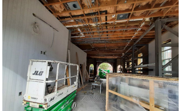
M/E/P rough-ins are almost complete on the ground floor. The crate in the foreground holds part of the elevator, which is being installed now. View from SE corner of building.
