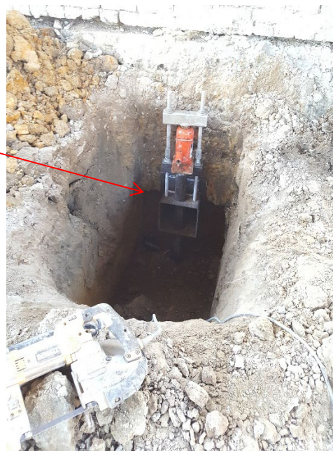
Temporary shoring bracket installed under existing foundation to allow excavation for new foundation.
