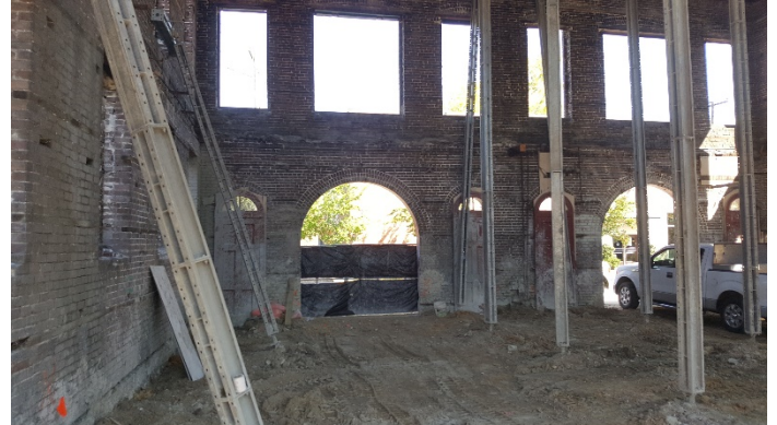
Installation of interior micropiles and temporary shoring complete.
