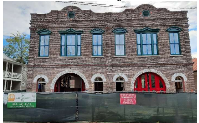
Cannon Street (north) elevation. First coat of paint has been applied to the windows. Tin headers and gable vents will be painted white. Colors based on historical evidence on site.
