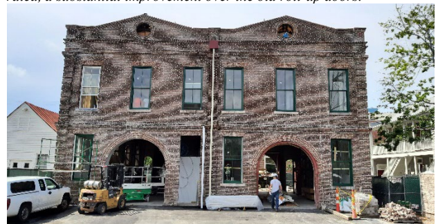
A view of the rear yard. Some of the windows have been trimmed out and painted. New wood doors will be placed in the arched opening.
