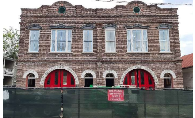
Cannon Street (north) elevation. New personnel door frames with transom windows have been installed.
