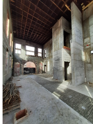
New concrete slabs have been placed, and include replica horse tracks along the center and where the old stalls would have been.
