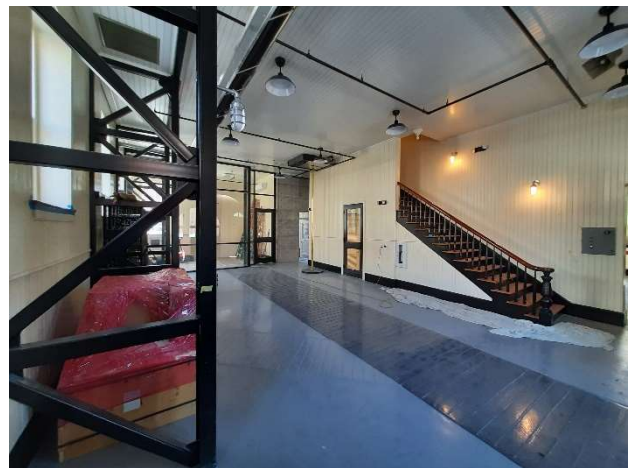
The other bay, viewed from just inside the main entrance. The historic handrail has just received the final coat of antique oil finish.
