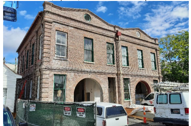
A view of the rear yard. The first of the replacement louvers has been installed in the west gable.
