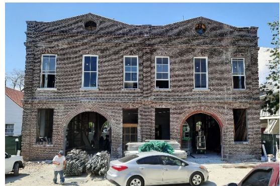
Masons continue repointing the lower portions of the building. Windows are being installed upstairs.
