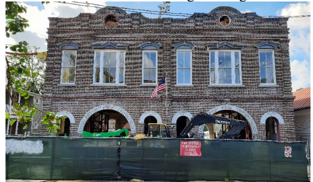
Cannon Street (north) elevation. The original decorative window headers have been cleaned, repaired, and re-installed. To be painted soon.
