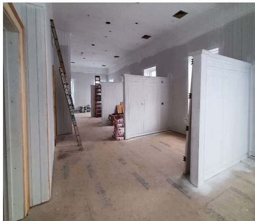
Bunkroom viewed from the front. Divider walls include doors from the old beadboard gear lockers.
