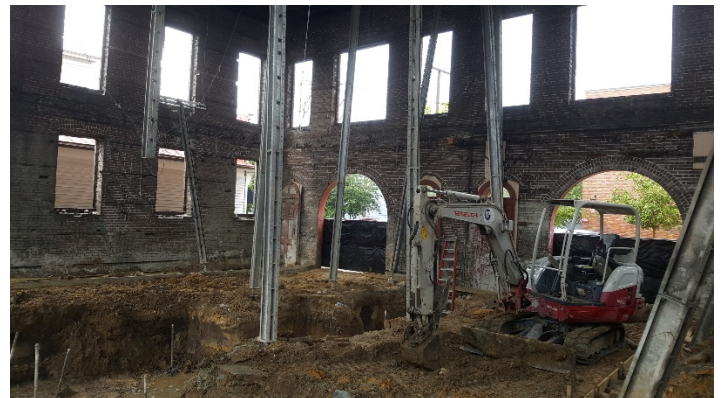
View from SE corner of interior towards Cannon St. showing the center wall foundation. Elevator pit will be in the bottom left corner of image.
