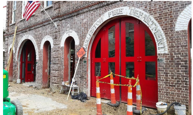
Cannon Street (north) elevation. The new bay doors are in place. Fire Engine 106 will be behind the closed door, and the open bay door is for the Battalion Chief vehicle.
