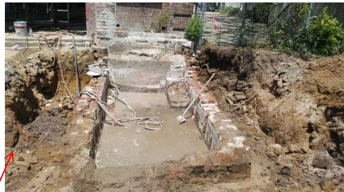
Large cistern (abandoned, approx. 2,000 gallon capacity) uncovered at the SE corner of structure. Originally provided water to steam boiler inside rear corner. A smaller cistern (approx. 750 gallon capacity) was uncovered at the SW corner. After comparing the two, it appears that the structure pictured was enlarged after the original construction.
