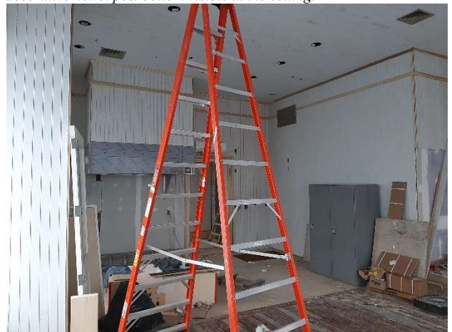
A view from the NE corner on the second floor, in the Day Room and Kitchen area. Salvaged Heart Pine floors have been laid in this room, the Study, and the Battalion Chief's quarters. The kitchen area will have quarry tile.
