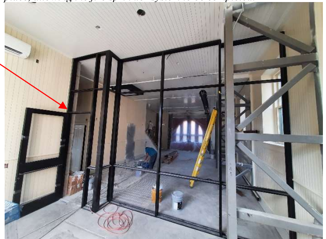
View of the smaller east bay from the SE corner. The black storefront will separate the exercise room from the Battalion Chief's vehicle bay. Reconstructed stairs are visible in the background.
