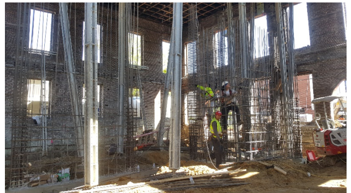
View from NE corner of interior towards fire tower, showing the center wall foundation. Elevator shaft rebar on the right side of image.
