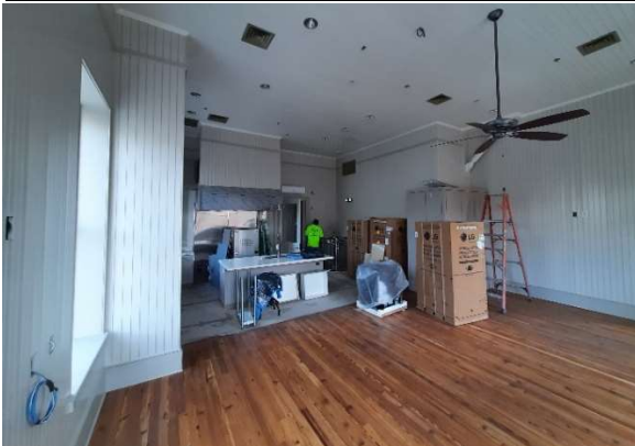
Day Room and Kitchen area. Countertops are in place and the trim-out of the M/E/P and FP systems is ongoing. The heart pine flooring in this room is original to the building.
