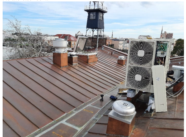
View of the copper roof towards the south. Final testing and balancing of the HVAC equipment is wrapping up. This roof system should last at least 75 years.
