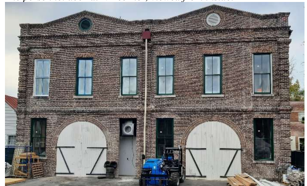
A view of the rear yard. The new arched doors are being fitted into place. These replacement doors are constructed of Sapele and marine plywood, assembled with a vacuum bag.
