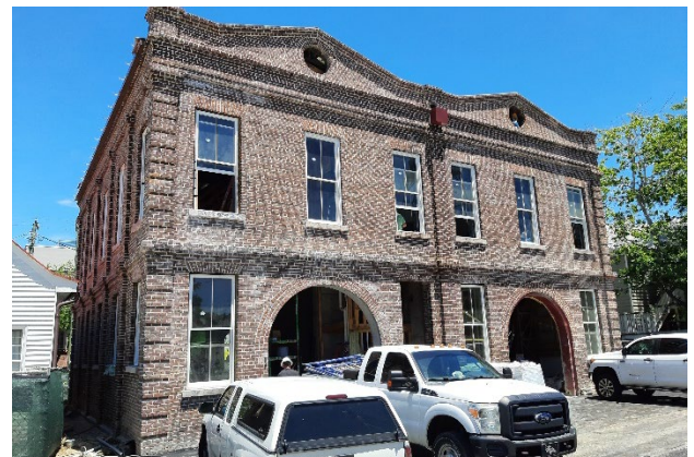
Repointing is complete except for touch-ups. Reproduction gable vents will be installed in the round openings at the top (front and back).
