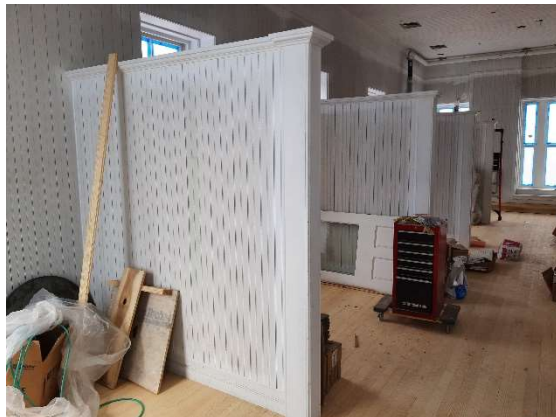
Bunkroom viewed from the rear. This face of the divider walls will be covered by three personal lockers at each bunk location. This room and several others have new heart pine flooring.
