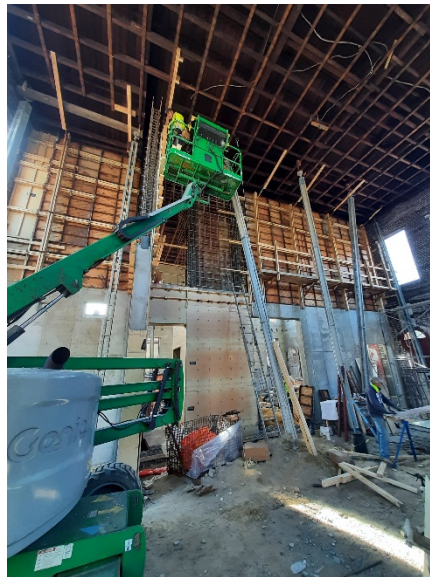
View of new center wall from east side, rear corner. This wall is a key part of the seismic improvements. Some of the new concrete will be exposed, and some hidden behind historic beadboard.
