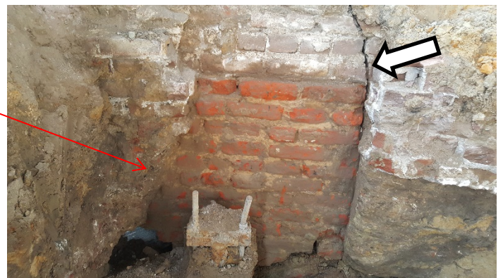
A brick structure remnant was found embedded in the foundation near the SW corner. Based on the materials removed from the soil on the outside of this wall, it is assumed to be an old privy pit (ca 1840). The manner of construction likely caused the cracking and settlement that exists in this corner of the station (the crack noted goes thru the wall).
