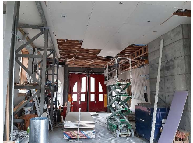
A view of the main apparatus bay (NW corner). Fire-rated gypsum board being installed on the ceilings will be covered by beadboard.
