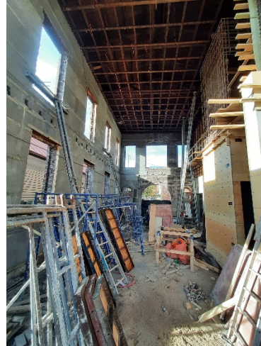
New center wall (R) is heavily reinforced concrete. Existing brick is being strengthened w/ fiber-reinforced stucco. West side view.
