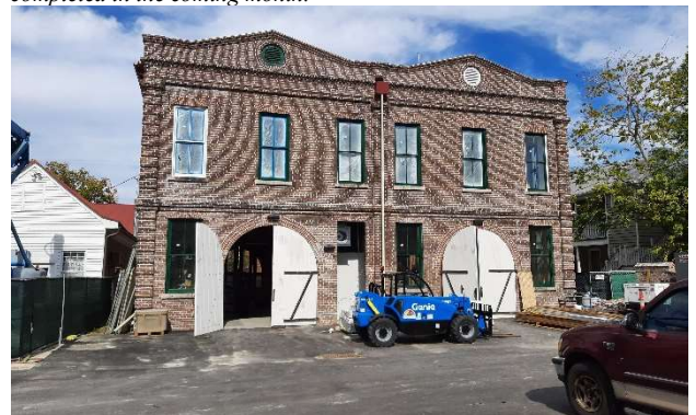
A view of the rear yard. The new arched doors are operational. The doors on the right will be fixed in place, but the doors on the left will allow the apparatus to roll into the rear yard to be washed.
