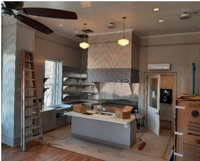
Day Room and Kitchen area. Stainless steel backsplash and open shelving has been installed. Final trim is underway. One of the new brass firepoles is visible beyond the refrigerator boxes, wrapped in blue plastic.
