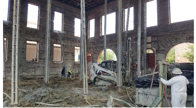
Injection-grouted micropile installation underway
