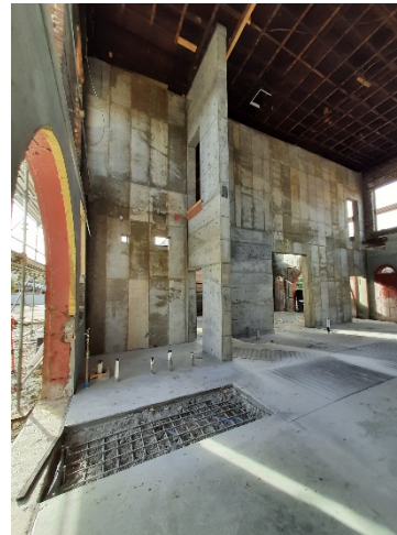
View of new center wall from east side, rear corner. The new floor is complete except for two locations where pieces of the original 'artificial stone' floor will be inset into the concrete.
