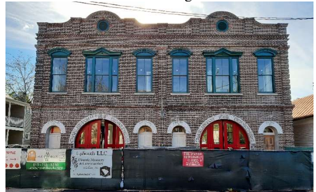
Cannon Street (north) elevation. All doors are in place, including a salvaged door at the NW corner. Driveway apron replaced and asphalt repaired (hidden by fence).
