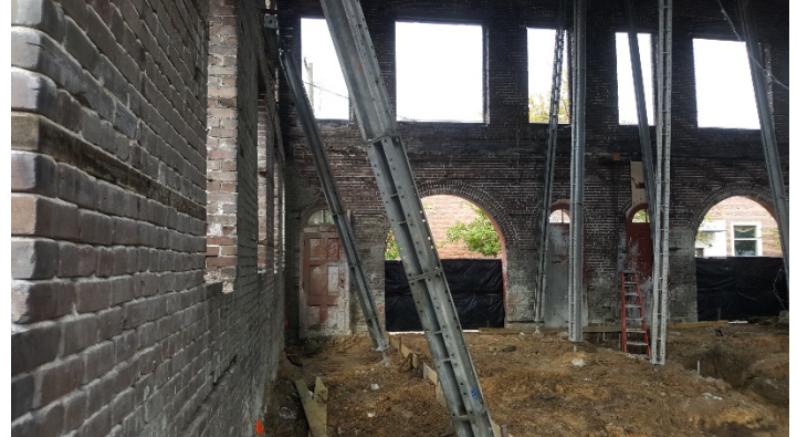
Excavation for new center wall foundation underway.
