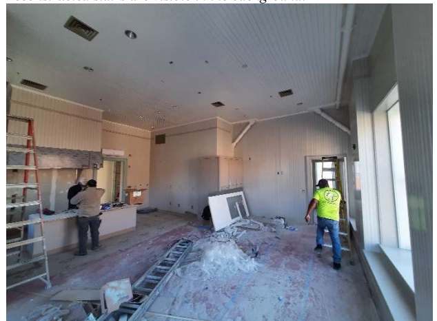
A view from the NE corner on the second floor, in the Day Room and Kitchen area. Cabinetry has been installed, walls and ceilings painted, and the trim-out of M/E/P systems is underway. Ceiling heights in this room and the bunk room match the original design. Other rooms on this floor have lower ceilings to allow room for mechanical equipment in the attic spaces.
