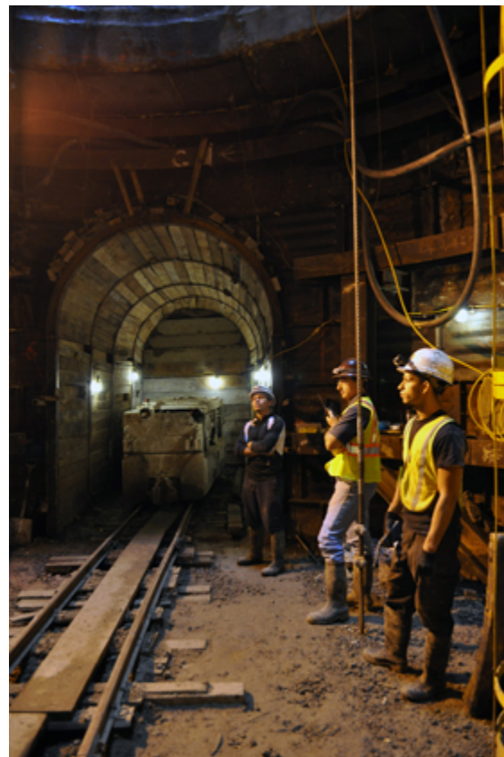
Market Street Drainage Project - Workers await supplies, which are lowered by a crane down the working shaft. The tail tunnel for the TBM (Tunnel Boring Machine) can be seen in the background.
