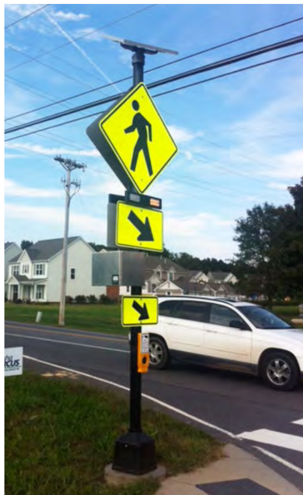
Rectangular Rapid Flashing Beacons (RRFB) utilize a warning yellow LED stutter flash light bar within the standard crossing sign assembly. They have proven an increased motorists yield rate versus other flashing beacon warning systems. They are especially useful at multilane crosswalks.
