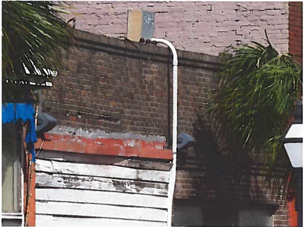
Figure 3 - Fractured upper facade.
