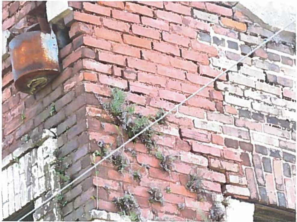
Figure 13 - Damage at northwest corner caused by expansion of corroding lintel.
