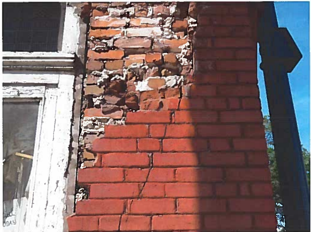
Figure 8 - Shear fracture in column.
