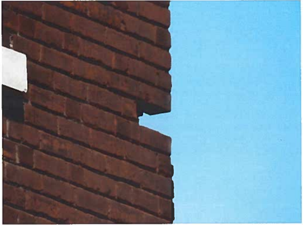
Figure 9 - Missing brick at third floor, corner.
