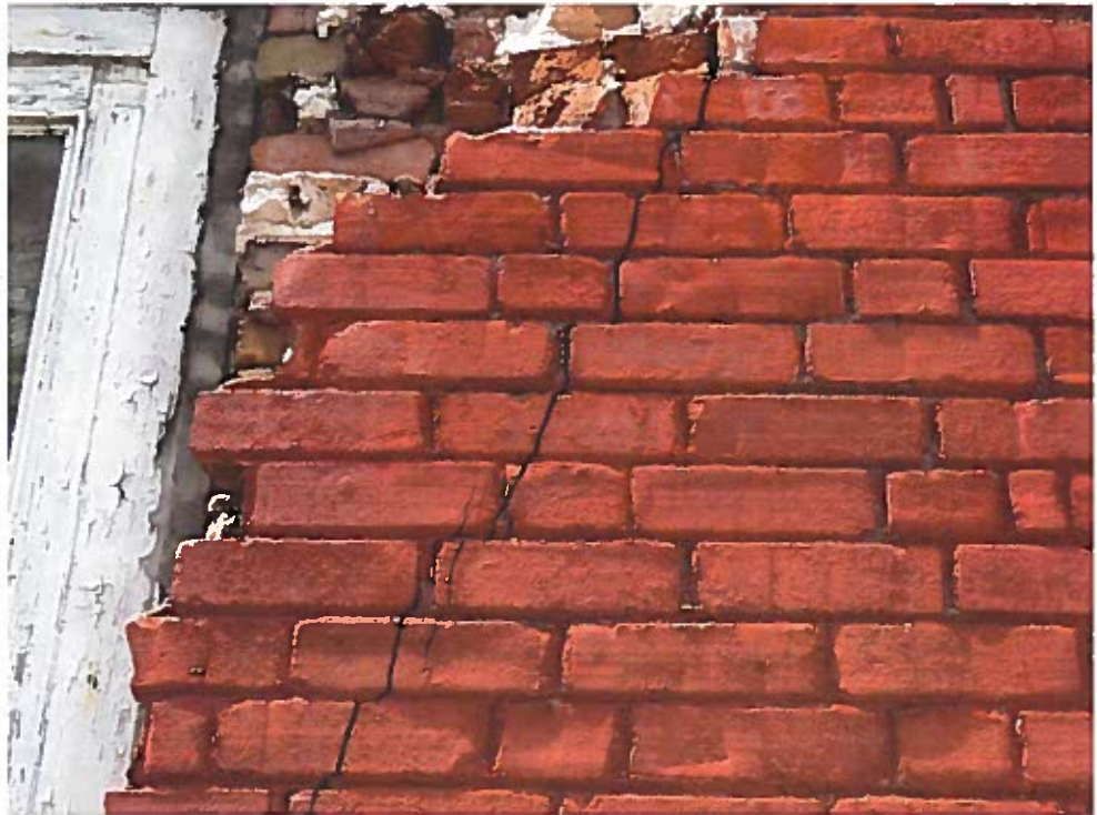
Figure 17 - Fracture in the same column.
