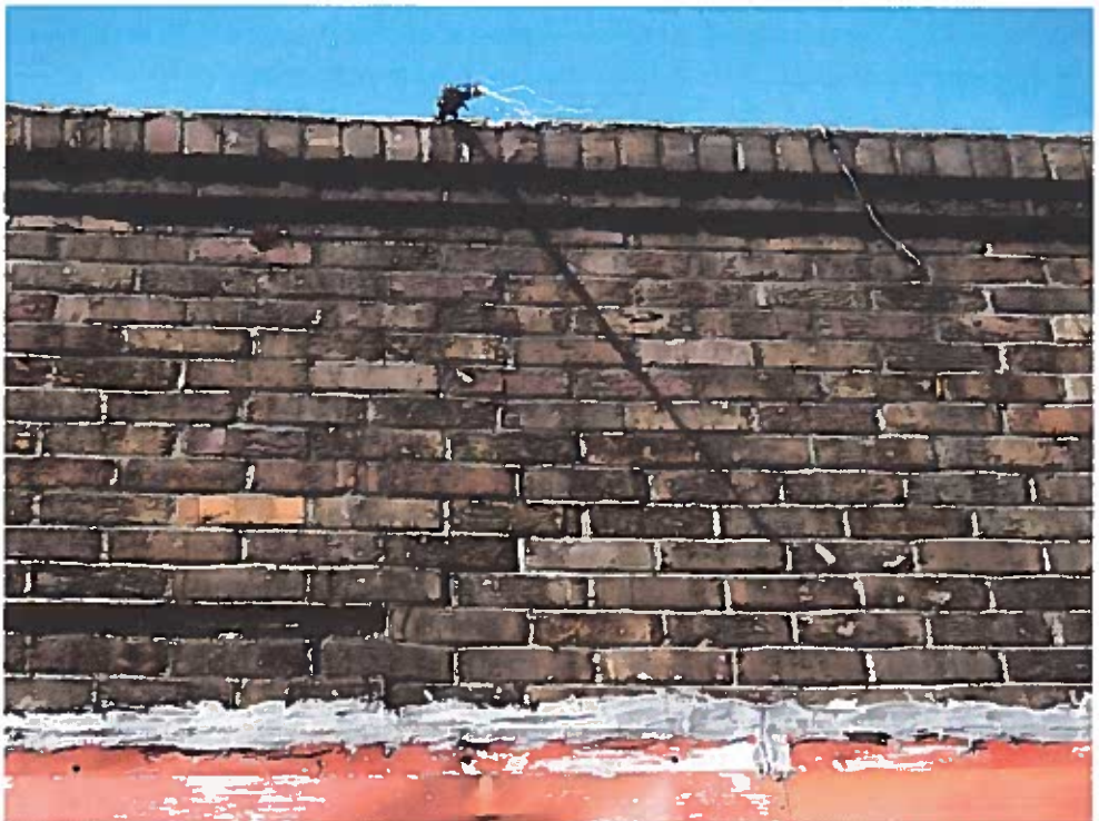
Figure 4 - Break in veneer at end of embedded steel beam.
