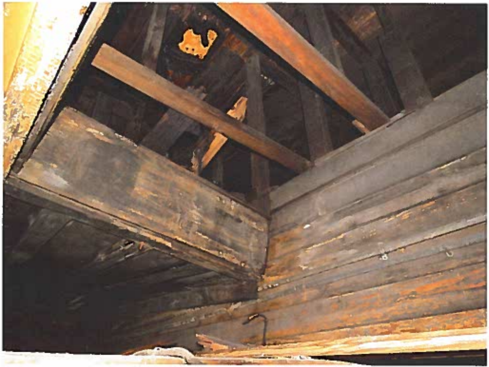
Figure 25 - Damaged roof structure in the same building.
