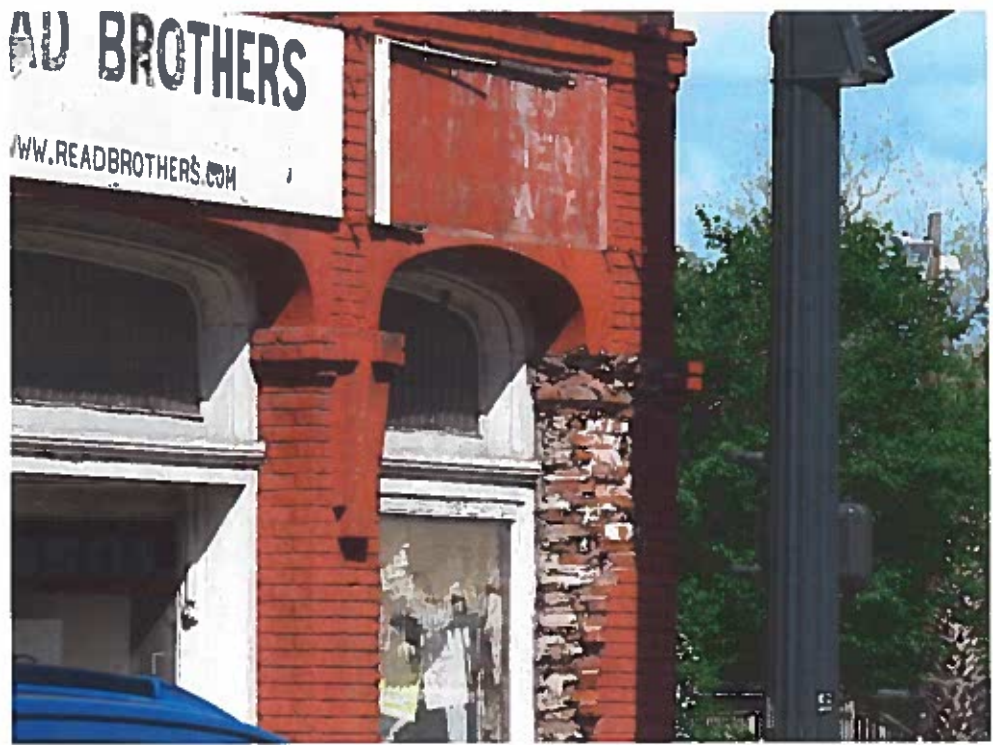
Figure 7 - Damaged corner column.
