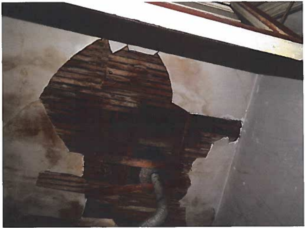
Figure 21 - Roof leak on the third floor.
