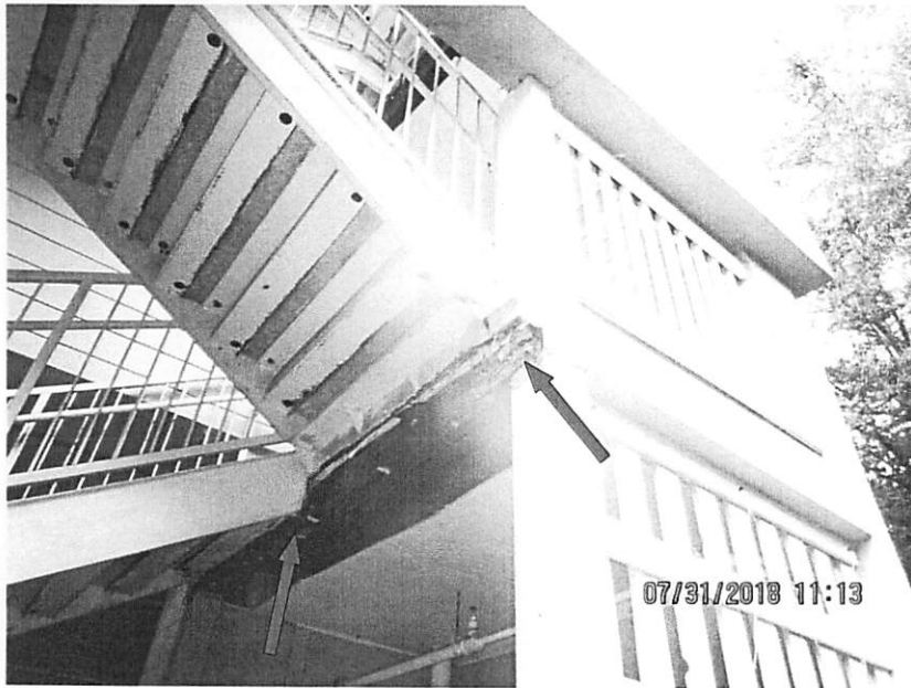
Photo 7 - Extreme beam damage at the second floor landing at Building A
