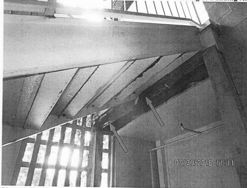
Photo 6 - Extreme beam damage at the second floor landing at Building A.
