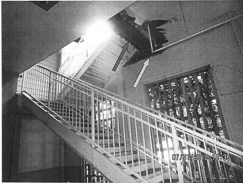
Photo 1 – Extreme beam damage at the intermediate and second floor landing at Building B. Extreme damage to surrounding structure at Building B (orange arrow)
