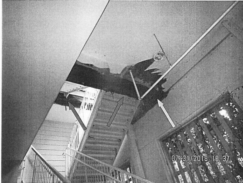
Photo 2 – Extreme beam damage at the second intermediate and second floor landing at Building B. Extreme damage to surrounding structure at Building B (orange arrow).
