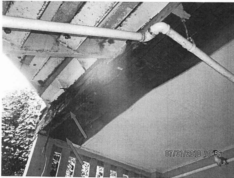
Photo 5 - Extreme beam damage at the second floor landing at Building A.
