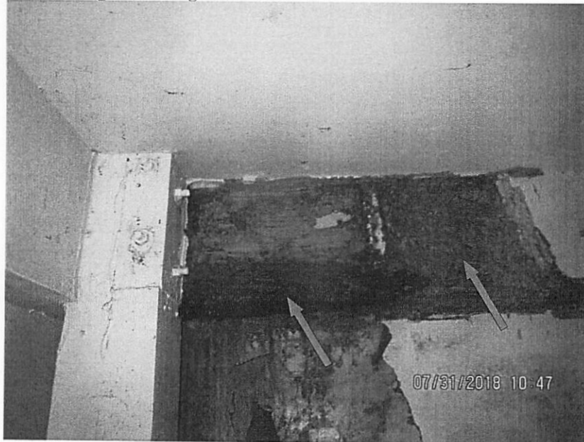
Photo 4 - Extreme beam termite and moisture damage at structure underneath heated space at Building B.
