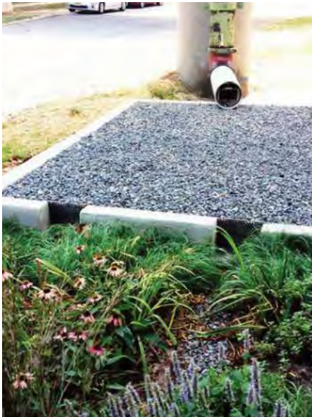
Retrofitted downspout
