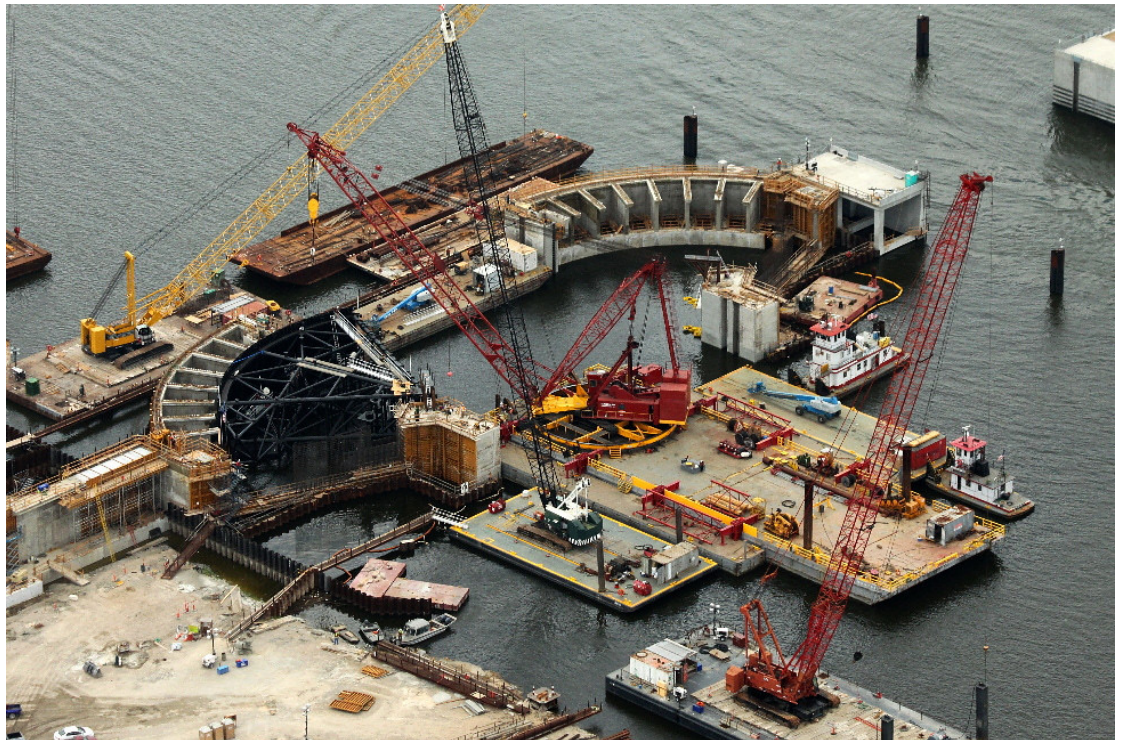
Sector Gate construction along the Inner Harbor Navigation Canal Lake Borgne Surge Barrier in Louisiana.
