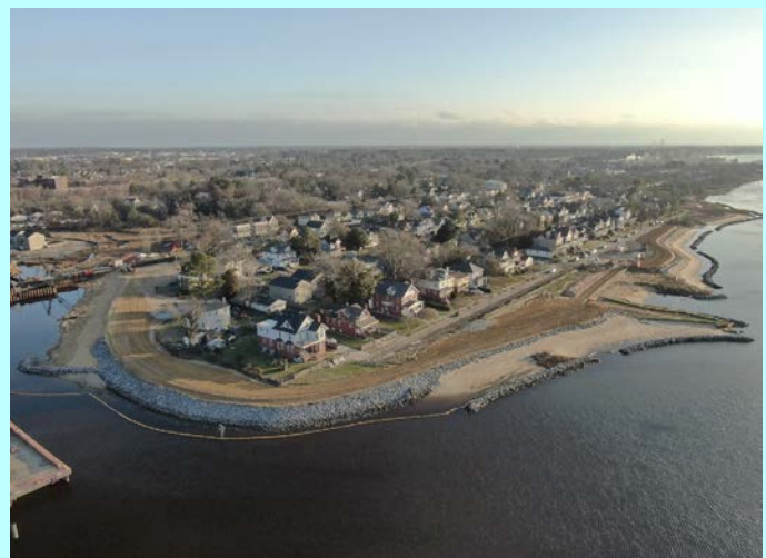
Living shoreline under construction in Norfolk, VA, 2020.
