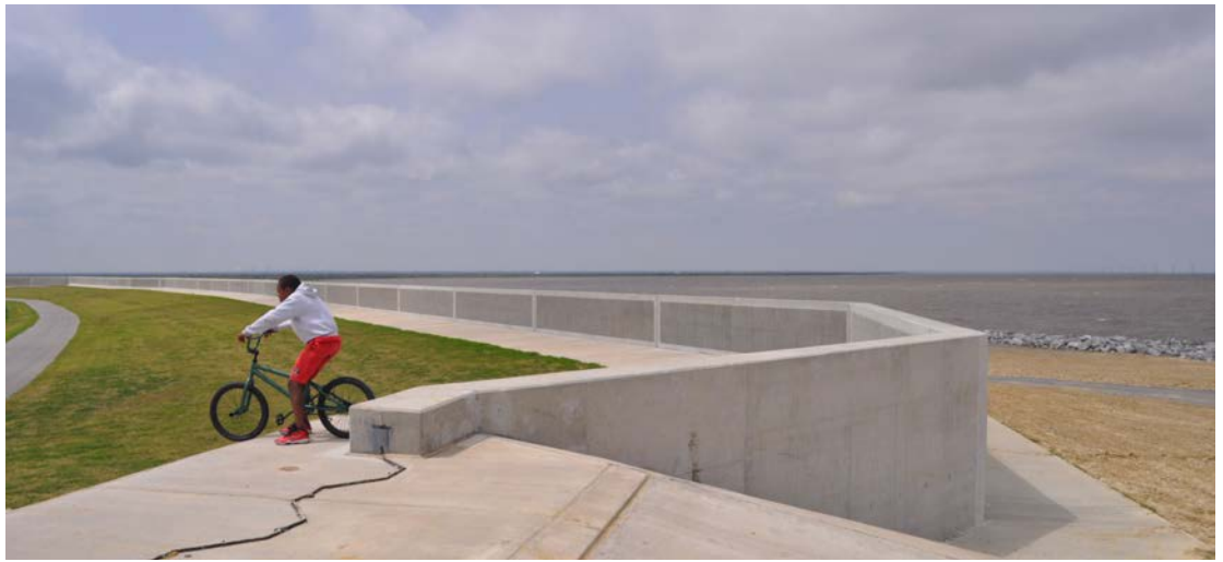
T wall structure in New Orleans along Lake Pontchartrain. Credit: Waggonner & Ball
