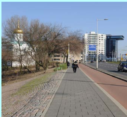
x70 year protection: Inside Rotterdam, levees are incorporated into the urban fabric as roads and inhabitable public spaces to subdivide the city for added flood resilience.
