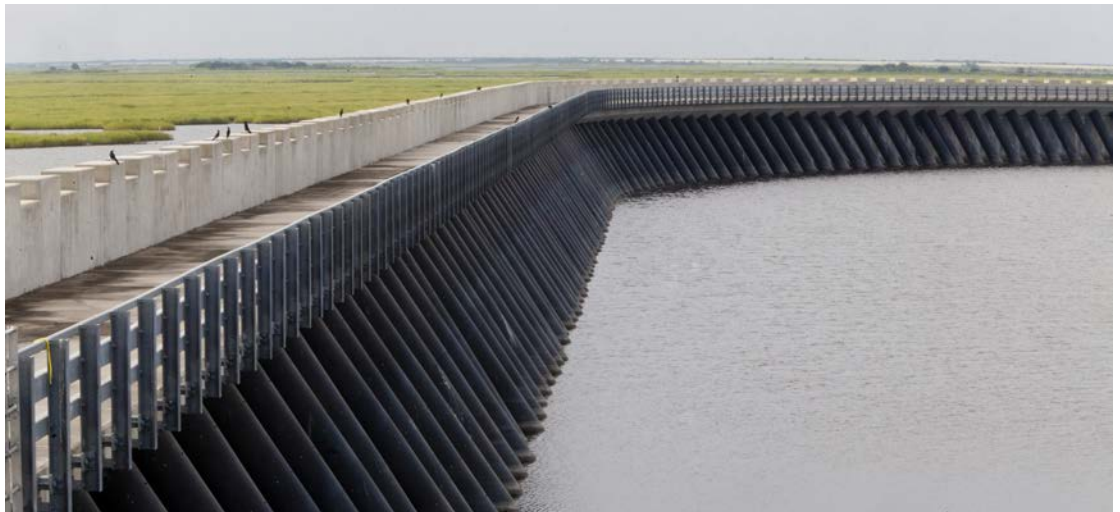
Combo wall structure part of the Lake Borgne Surge Barrier. Credit: Philip Gould Corbis
