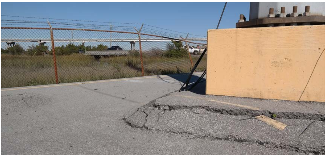
Subsidence at Columbus Terminal.
