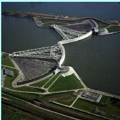
x100 year protection: The Maeslant Barrier, a Delta Works project outside Rotterdam, is the city’s first line of defense, closing to stop storm surges from the North Sea.
